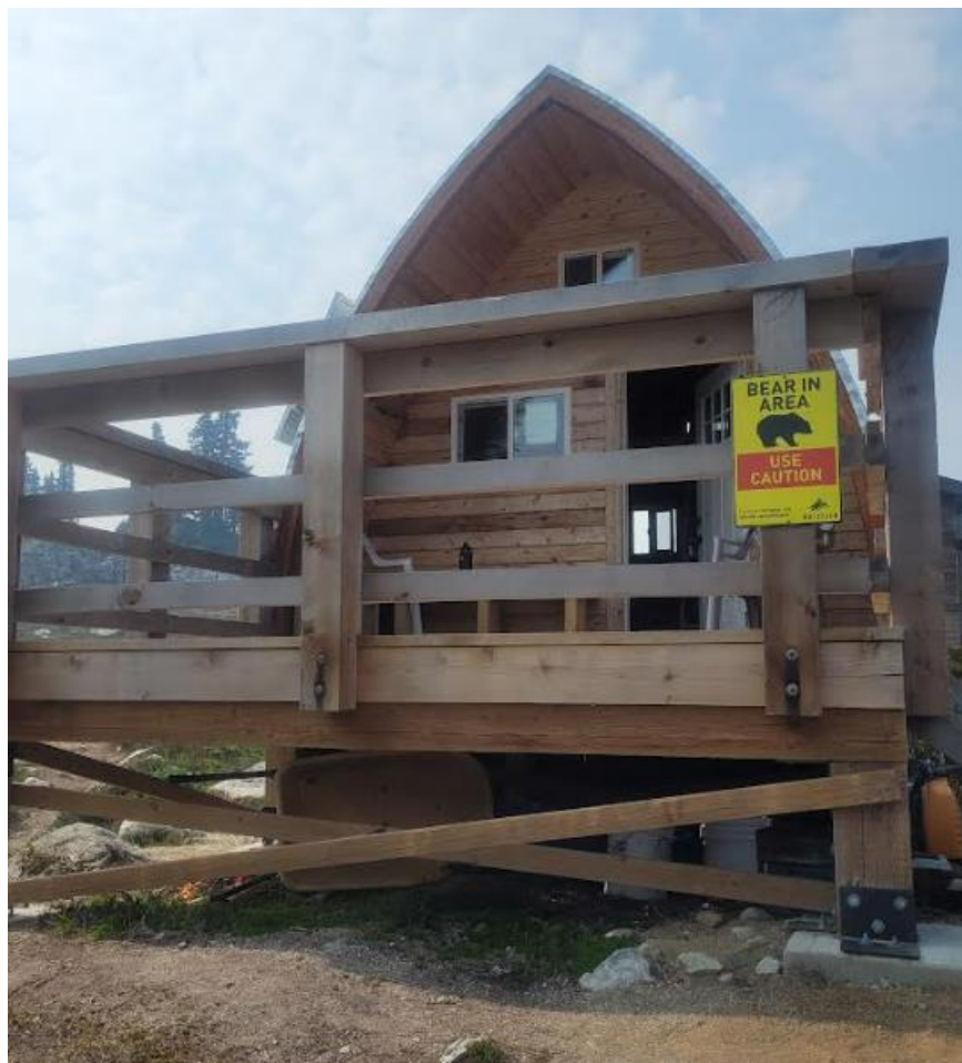
Figure 1: Newly erected signage
