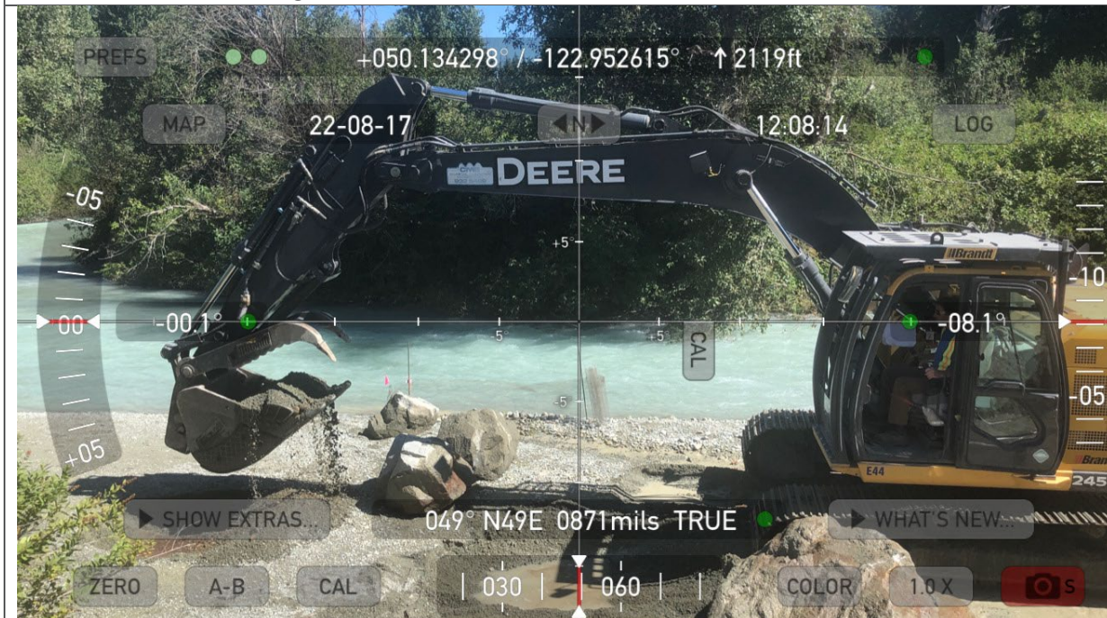
Photo 2: Gravel Bar #19 preparing for excavation. Fish net present for fish salvage.
