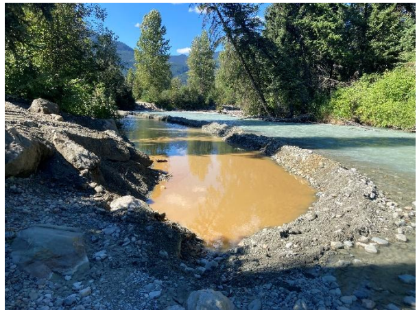
Photo 8: Looking north at the access ramp and constructed berm of Bar 17. August 22, 2022.
