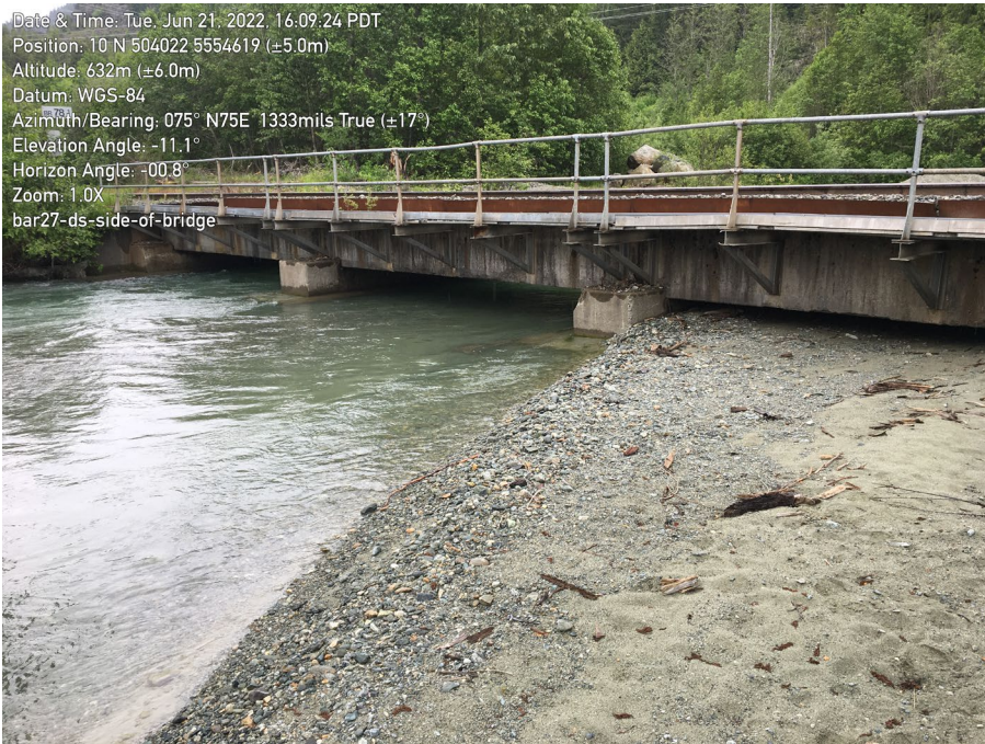
Photo 15: Gravel Bar #27 downstream side of CN railway bridge. Estimated gravel extraction volume = 442 m 3 .
