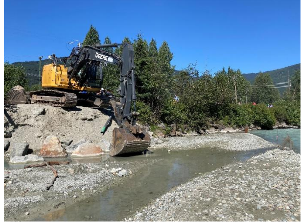
Photo 10: Excavator operator preparing the Bar 18 access ramp. August 17, 2022.
