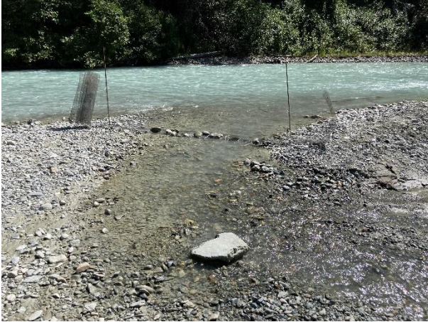
Photo 9: Installation of fish exclusion fencing at Bar 18. August 16, 2022.
