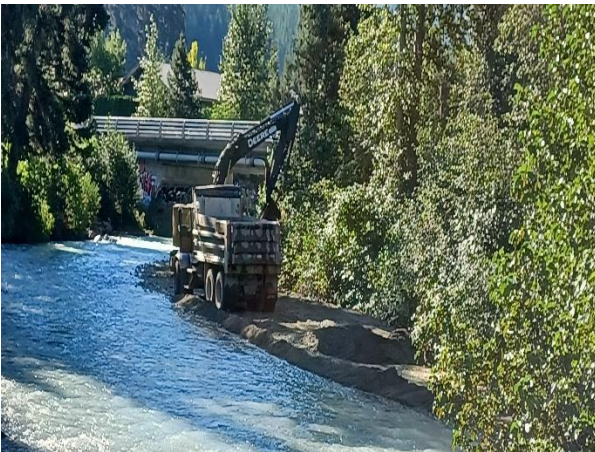
Photo 7: Excavation of Bar 17. August 22, 2022.
