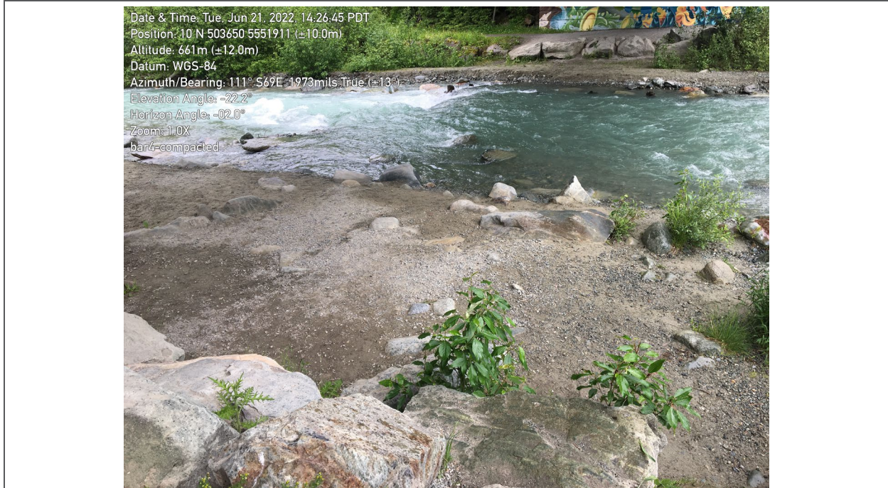
Photo 2: Gravel Bar #4 compacted. Estimated gravel extraction volume = 337 m 3 .
