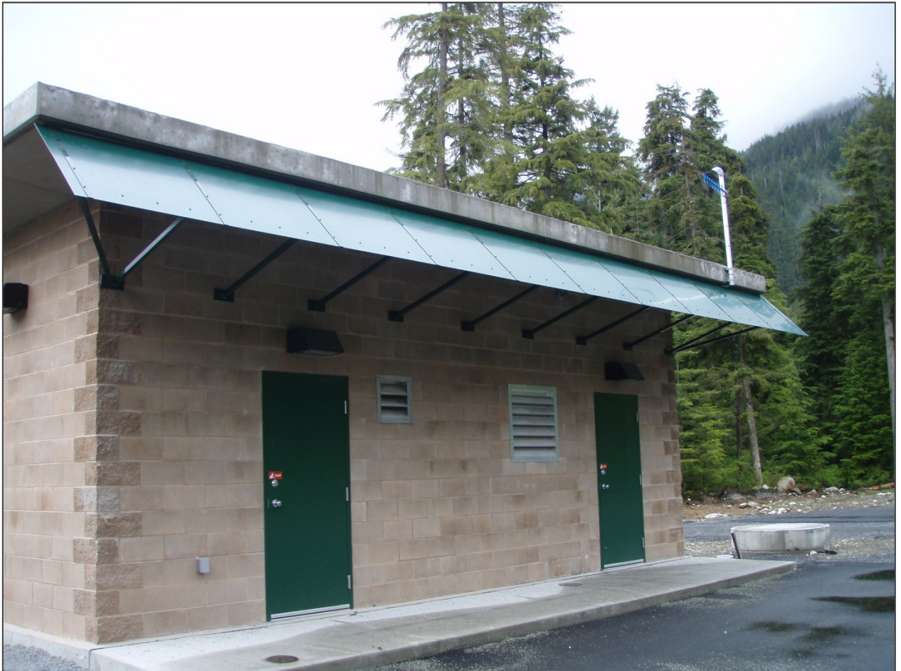
Figure 7-1: Cheakamus Crossing Pump Station
