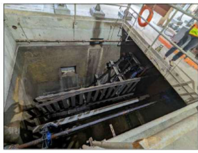
CROSS COLLECTOR MECHANISM AND FINGER BAFFLE
