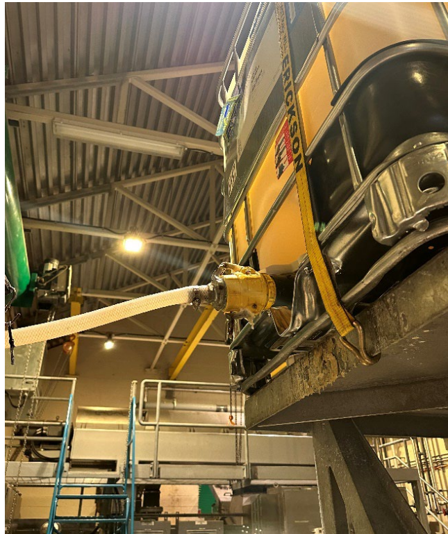
Figure 3: Polymer Tote Hose Line Hookup
