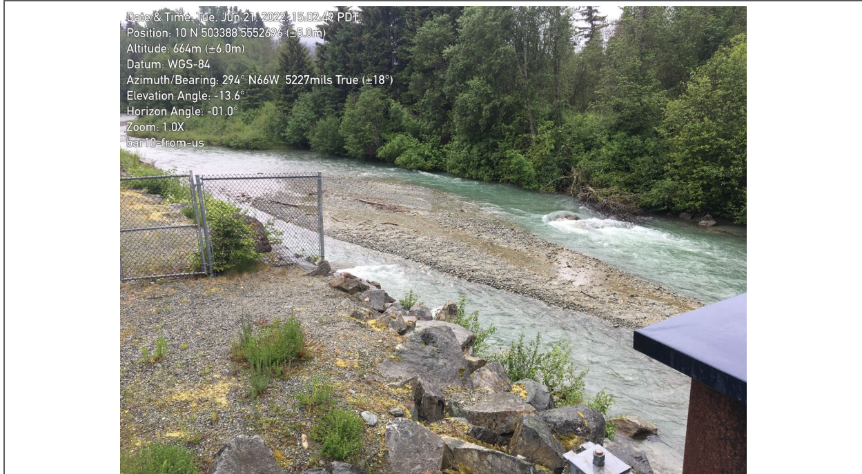
Photo 6: Gravel Bar #10 from upstream. Estimated gravel extraction volume = 764 m 3 .
