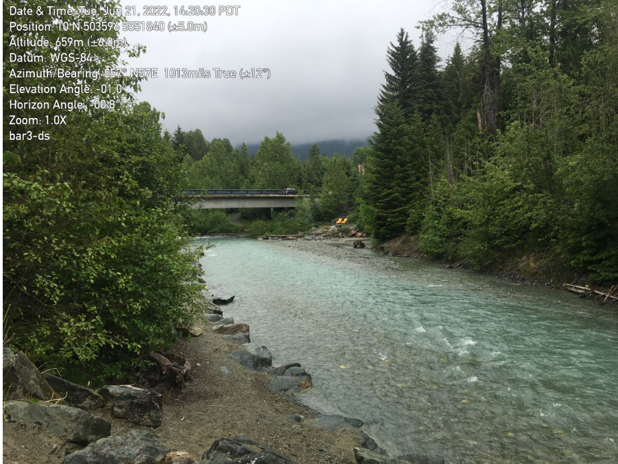
Photo 1: Gravel Bar #3 facing downstream. Estimated gravel extraction volume = 255 m 3 .
