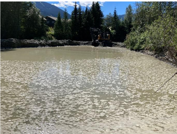
Photo 3: Excavation of gravel on Bar 15. August 16, 2022.
