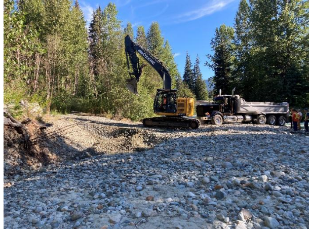
Photo 2: Constructing a ramp for Bar 15 access from Valley Trail. August 15, 2022.
