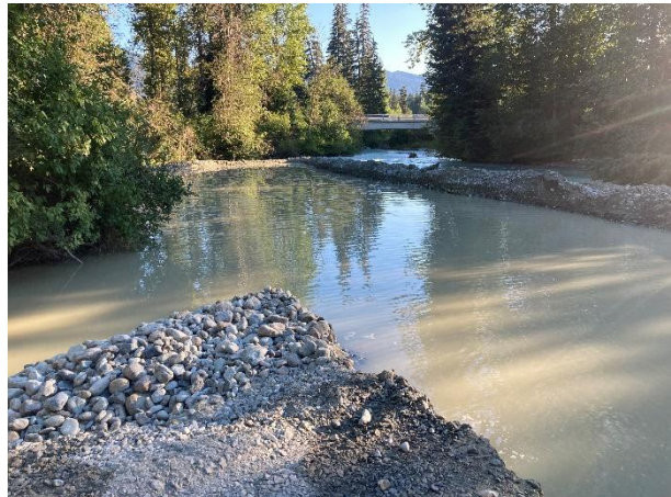
Photo 4: View of gravel Bar 15 following the excavation. August 17, 2022.
