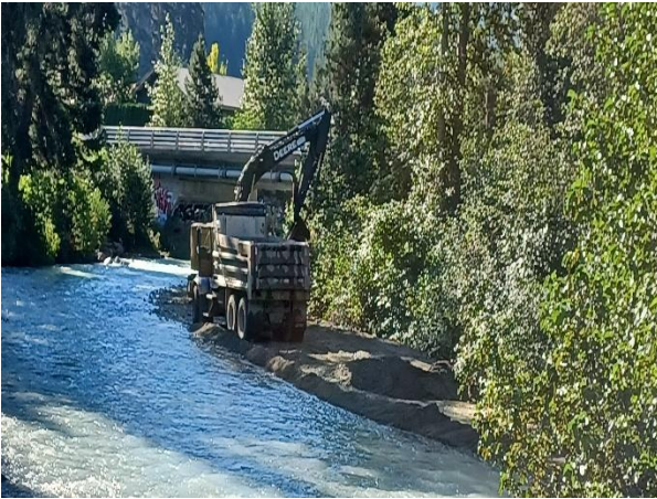
Photo 7: Excavation of Bar 17. August 22, 2022.
