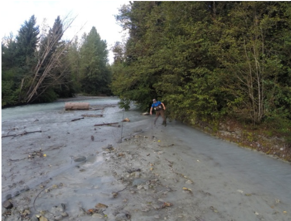
Photo 1: Isolation of side channel in preparation for wet crossing
