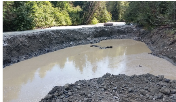
Photo 4: Isolation berm and partially excavated gravel bar.
