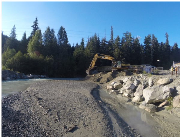
Photo 5: Constructing diversion berm with material from the left bank
