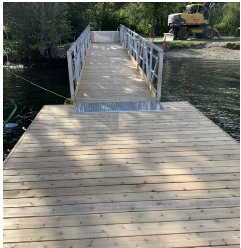
Image of Ramp to Dock transition
