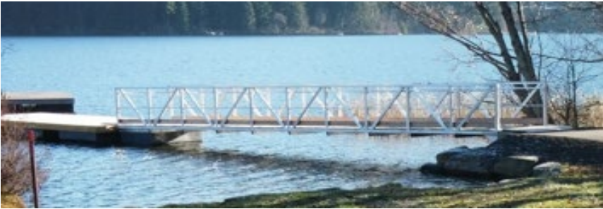
Image of Identical ramp and dock installed at Rainbow Dog Beach
